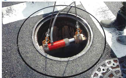
③ 仮蓋設置
